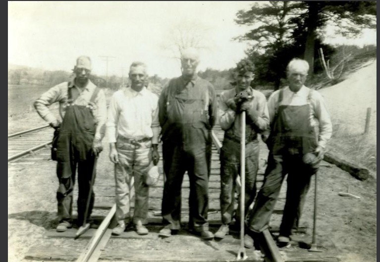
Section gang photo. One of the two men in the center not holding any tools is likely the foreman. The man on the left is holding a spike maul that is used to hammer spikes into the ties. The man second from the right (Theodore Mack of Webster) is holding a spike puller, a long tool with a forked end used for removing spikes. HHS collection.
